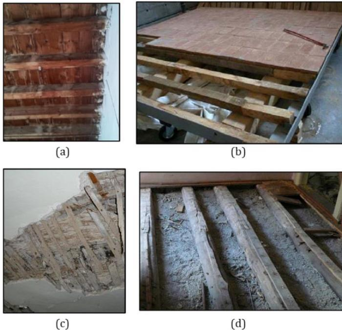
**Figure 10.1** — Diaphragm typologies: a) single straight sheathed diaphragm with squared timber joists; b) floor with clay tiles over joists; c)/d) floor built with the so-called “malta-paglia” (mortar-straw) technique, beneath and above views
